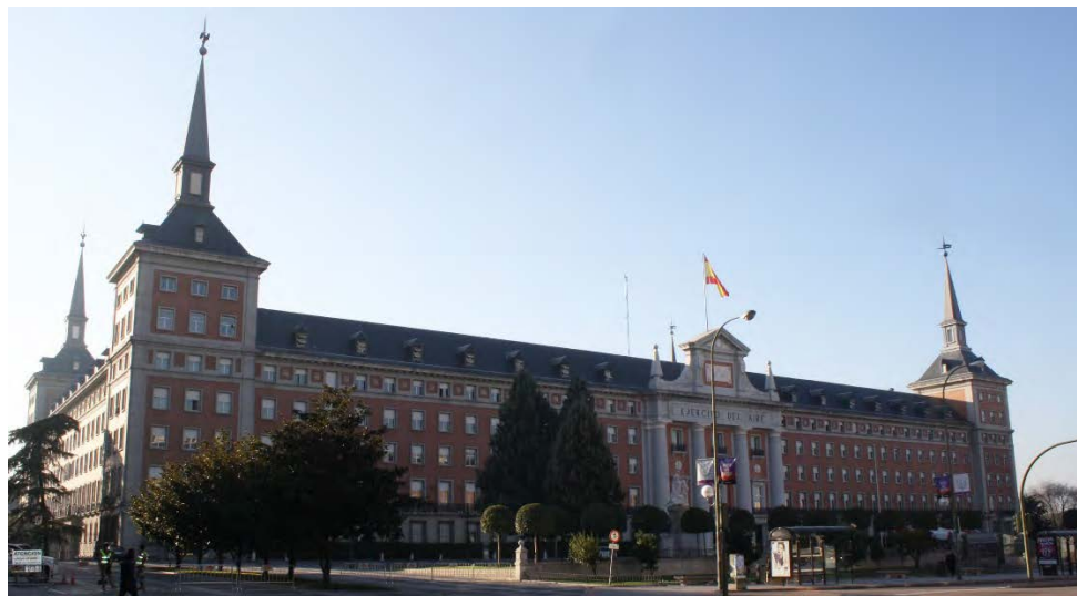
Figure 4. Headquarters of the Ministry of the Air, Luis Gutiérrez Soto, 1942-1958, Madrid. Photo by Emma López Bahut.
