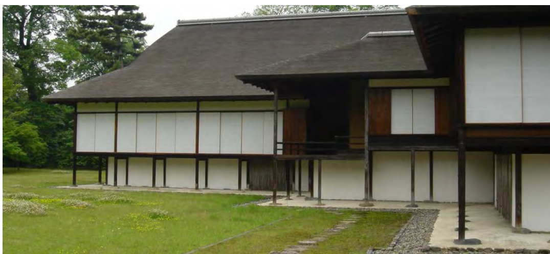
Figure 1. Katsura Villa’s shoin-zukuri buildings from left to right: Shin-goten, Chū-shoin and Ko-shoin, in the diagonal zigzag “flying geese” layout. (Photo by the author.)
