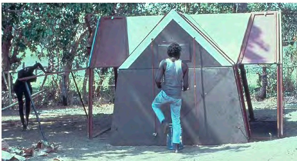
Figure 5. A Goorawin under construction at Aurukun, 1976. Photograph Mike Heppell.
