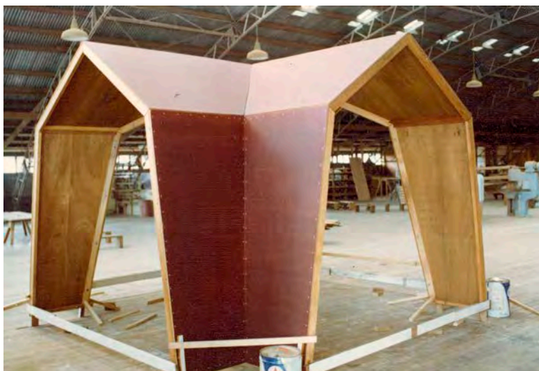
Figure 3. A cruciform Goorawin prototype without hinged walls. Photograph Mike Heppell (AIATSIS, HEPPELL.M02.CN).
