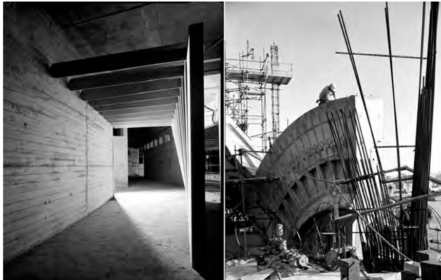
Figure 6. The 'beton brut' finishes of The Sydney Opera House, uncommissioned construction photographs, 1958-1964. (source of images: Mitchell Library, State Library of New South Wales and Courtesy Max Dupain and Associates)
