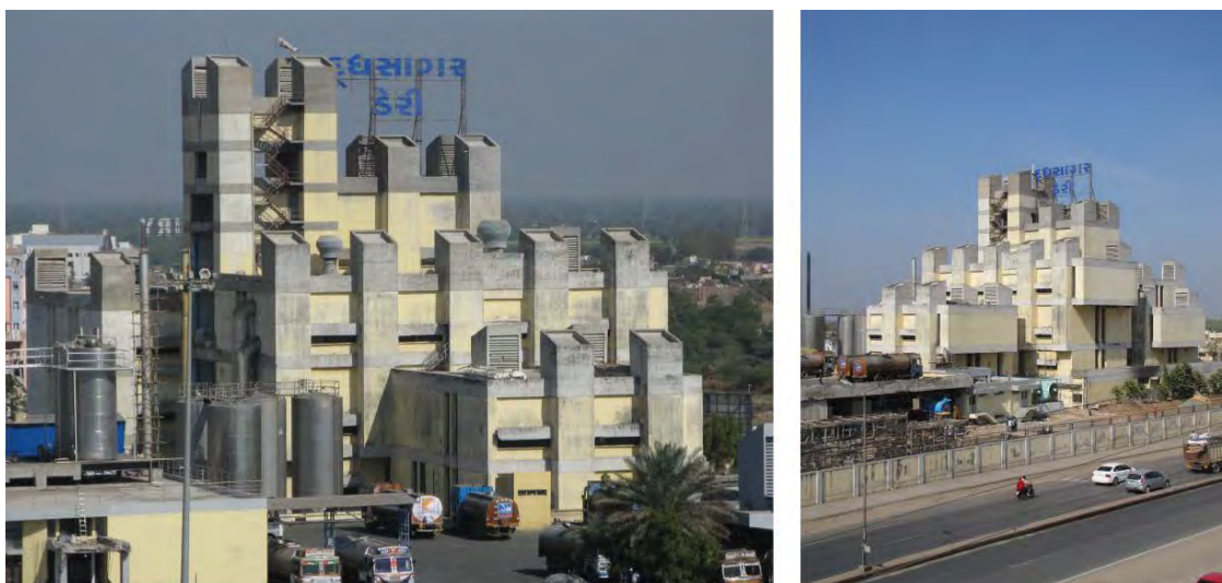
Figure 2 (left). Kanvinde, Dudhsagar Dairy, Mehsana (1970-73), Lattice of ventilation shafts and production units. [Photograph by author, 2011]. Figure 3 (right). Kanvinde, Dudhsagar Dairy, Mehsana (1970-73), Topographic composition. [Photograph by author, 2011].
