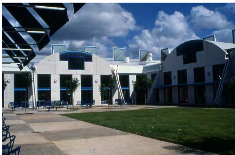
Figure 5. View of Watson’s Meadowbrook building from the courtyard: an array of square skylights line the crest of the roof, and demi-portico, demi-buttress downpipes, are positioned at regular intervals along the Eastern and Southern walls. (Photograph by Don Watson)
