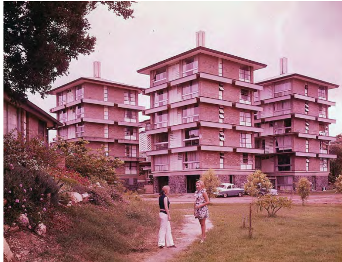
Figure 5. International House, University of Queensland, St Lucia, Queensland (1965-9) – architects: Fulton & Collin (Design Architect: Stephen Trotter). Source: University of Queensland Archives.
