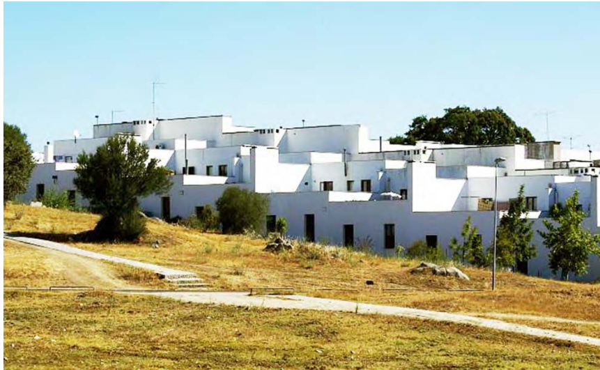
Figure 2. Malagueira housing, (Modified by Rahmatollah Amirjani, adapted from Photo pin, http://photopin.com/free-photos/malagueira ).
