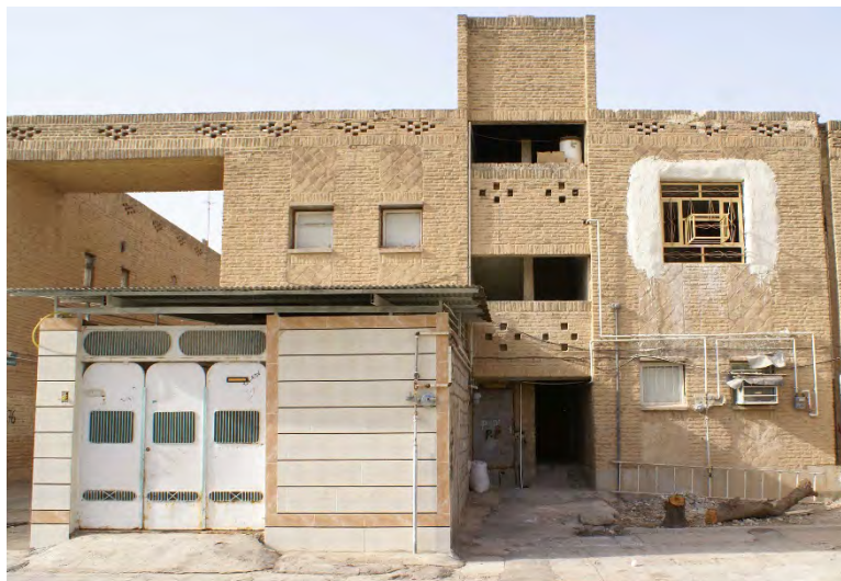
Figure 6. Shushtar New Town, the installation of new gas pipes and cooling system (Photograph by Rahmatollah Amirjani, 2012).
