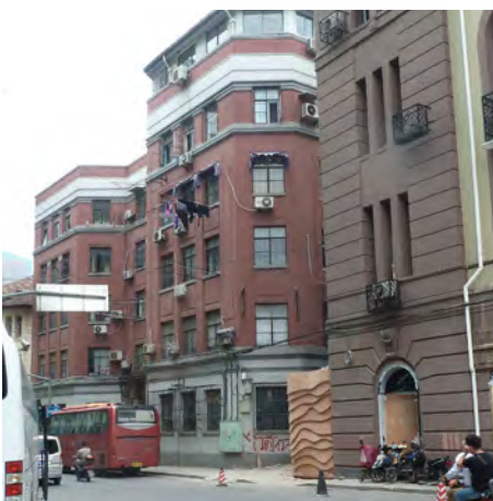
Fig. 2 YMCA National Headquarters Shanghai, Shattuck & Hussey, architects, 1921. Photograph by Anne Warr, May 2015.
