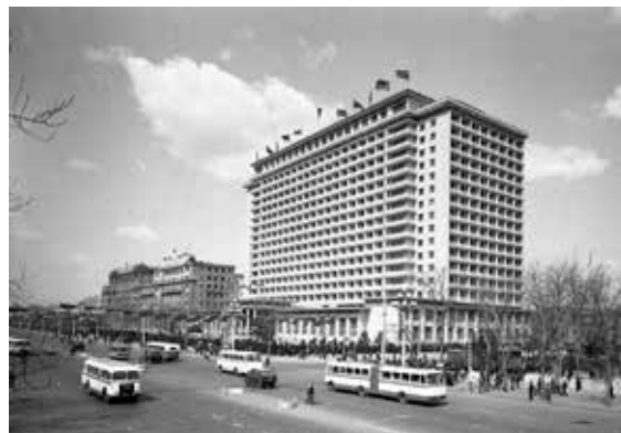
FIGURE 6 Beijing Hotel East. Source: courtesy of BIAD.
