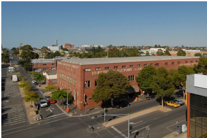
Figure 9. Woolstore, 20-28 Brougham Street, Geelong (Photograph by the authors, 2022).
