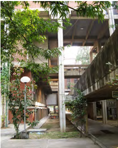
Fig. 2 IITK double level corridors through library building. Photograph by Prajakta Sane, 2011.
