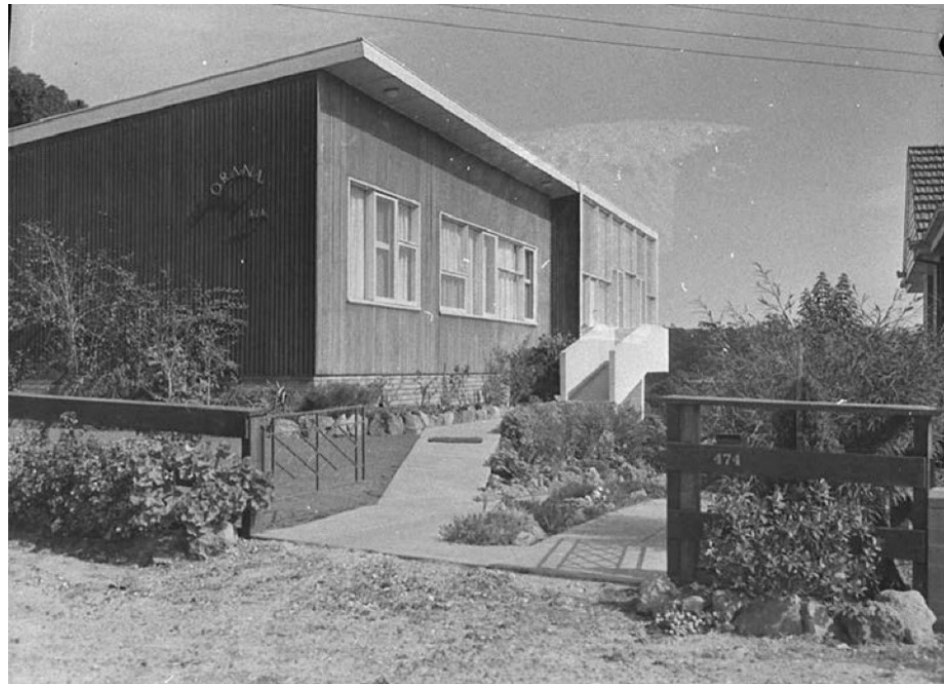
Figure 2: 'Orana', Adamstown Heights, Newcastle, NSW. Source: State Library of New South Wales, Home and Away – 28233 (photo: 16/8/1955).
