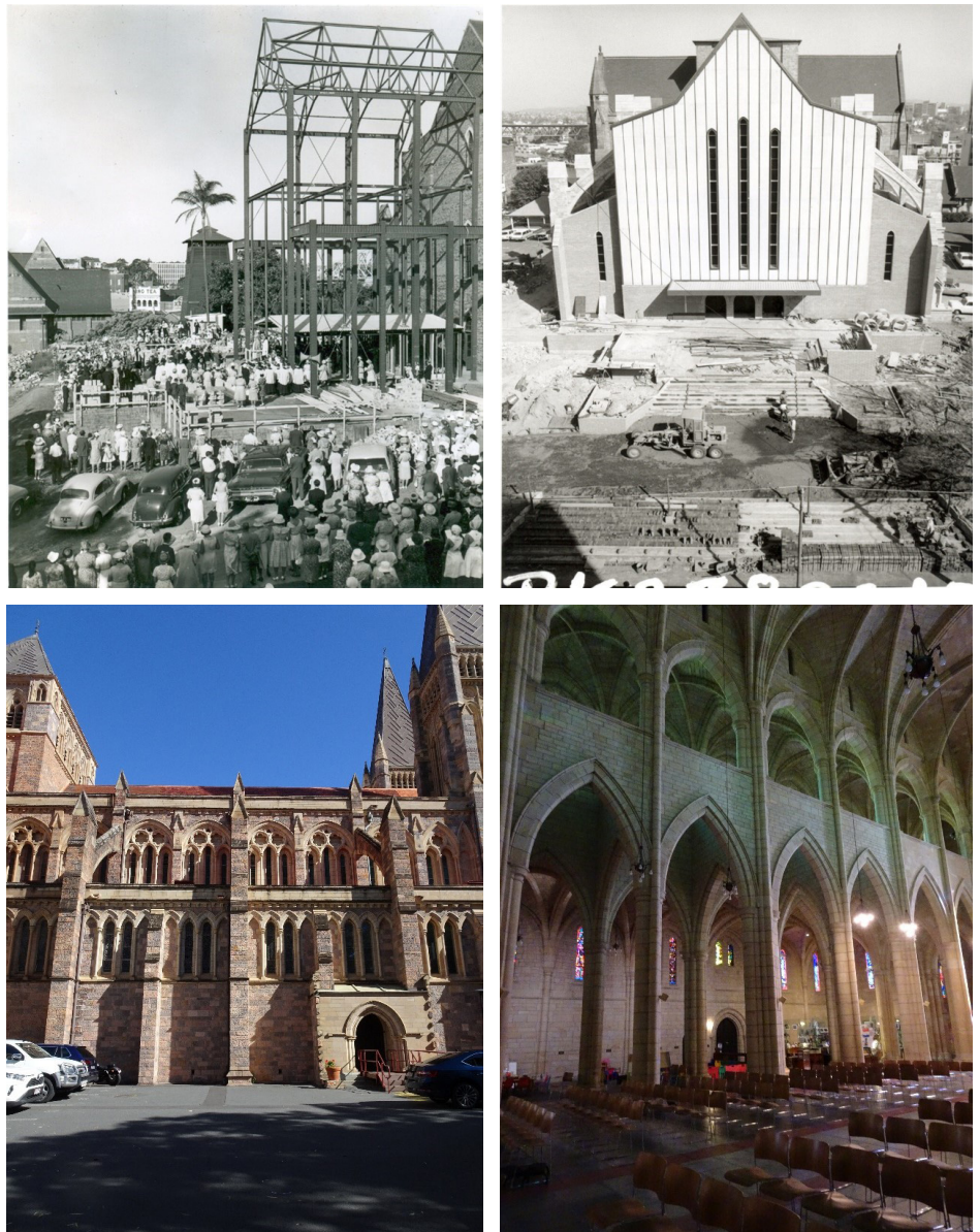
Figure 3: St John's Church of England Cathedral, Brisbane, War Memorial extension works (1910 stage I, 1968 stage II extension), by Conrad, Gargett and Partners. Top Left: November 21, 1965 photograph of steel framing, photographer unknown. Top Right: 1968 photograph of temporary west wall, photographer unknown. https://www.anglicanchurchsq.org.au/archives/cathedral-exhibition accessed June 26, 2021. Reproduced with the permission of the Records and Archives Centre, Anglican Church Southern Queensland. Bottom: Photographs of the stage II bays, by Lisa Daunt 2021.
