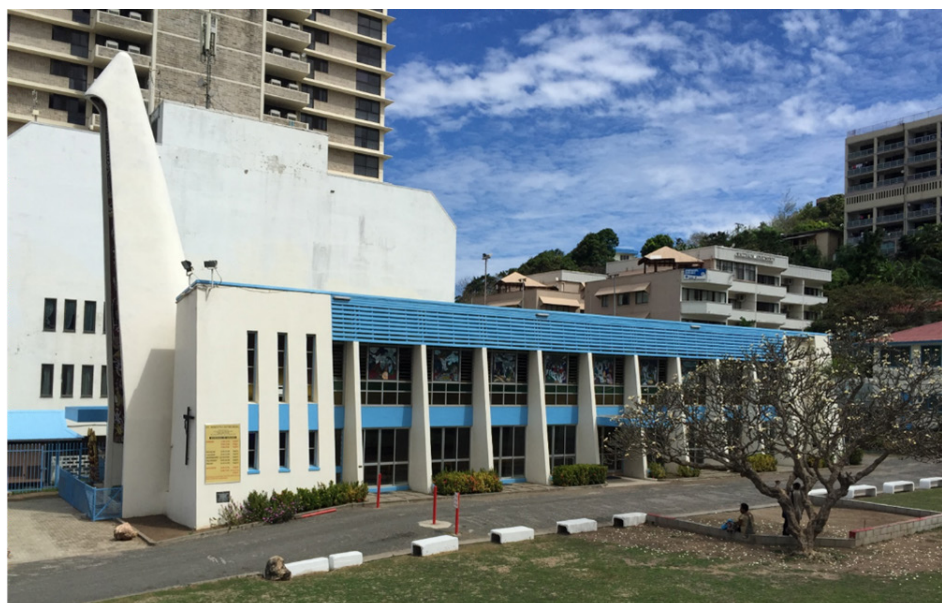
Figure 6: St Mary's Cathedral, Port Moresby, PNG (1969), by A. Ian Ferrier, in association with John R. Wild. Top and middle: The revised and built design's street elevation and floor plan, June 1968 drawings Ferrier Baudet Archive, courtesy of Catherine Baudet Bottom: Exterior photograph, by Dr. Stephen Long, 2016.
