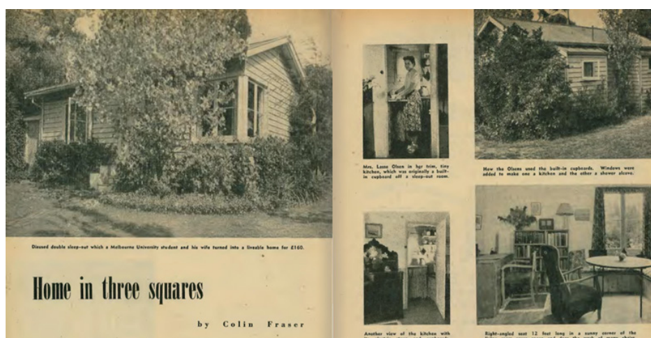
Figure 18: This sleepout converted into a flat in 1943 was still in use in 1948, Australian Home Beautiful , July 1948.
