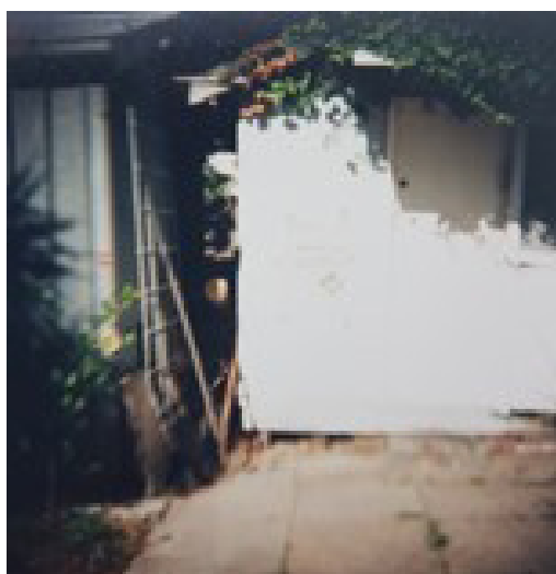
Figure 17: Sleepout of fibrous cement sheet, roofed in corrugated cement sheet and lined with Caneite in Brunswick, Victoria, possibly a WWHT sleepout. Photograph from a private collection.
