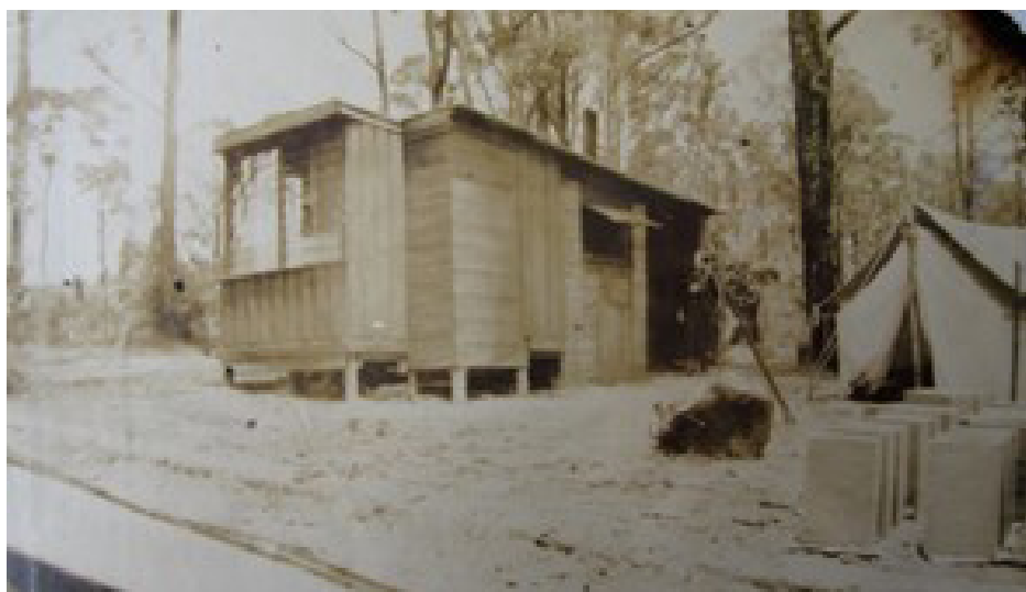
Figure 19: Timber sleepout used by Mrs Eager (pictured) while her sons David and Will slept in the tent on the right as they built a house for David and his fiancée Daphne in Wandin, Victoria 1947-8. Photograph collection of the Eager family.
