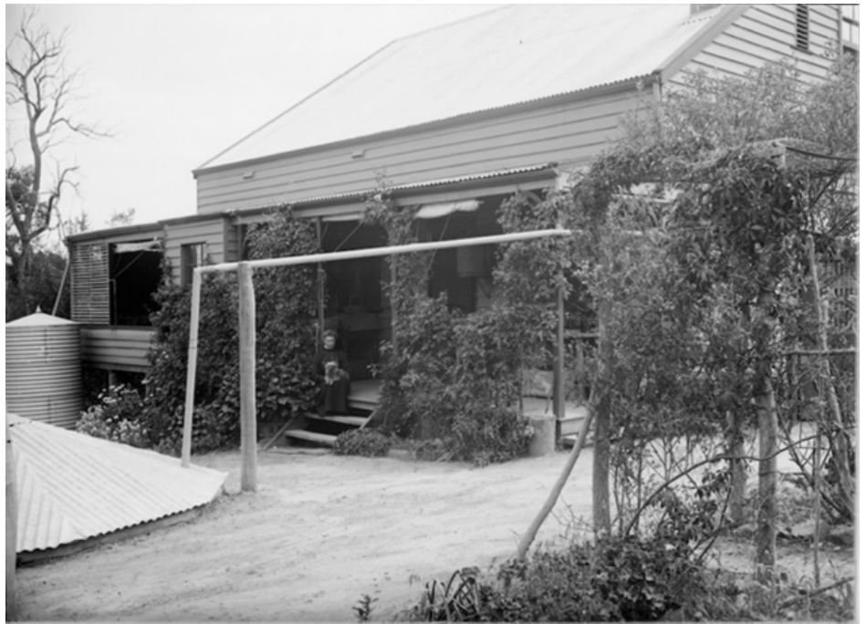
Figure 9: View of the back of a farmhouse with sleepout, 1910-18, Albert Jones, photographer, collection of the State Library of Victoria.
