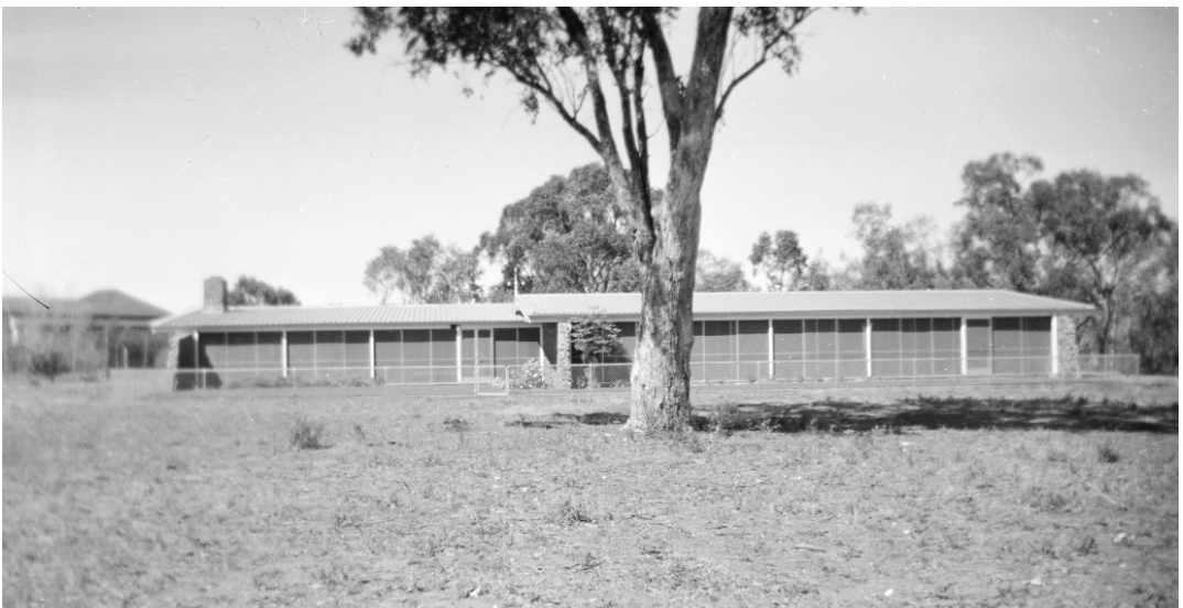
Figure 1. John Dalton Architect and Associates, “Morocco” homestead, St George, Darling Downs, (1963). Image shows new homestead in the foreground and the original house shown behind. (Photograph courtesy of Noela Wippell.)
