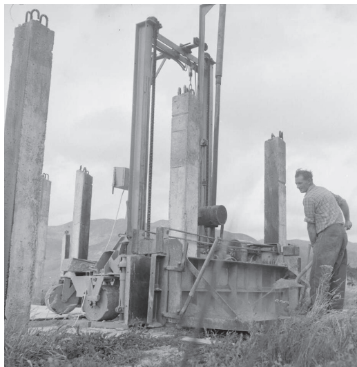
Figure 2. Photographs of the Terracrete system. Photos from "Clay-Cement Revives Ancient Building Styles," Evening Post (Wellington), February 2, 1958.
