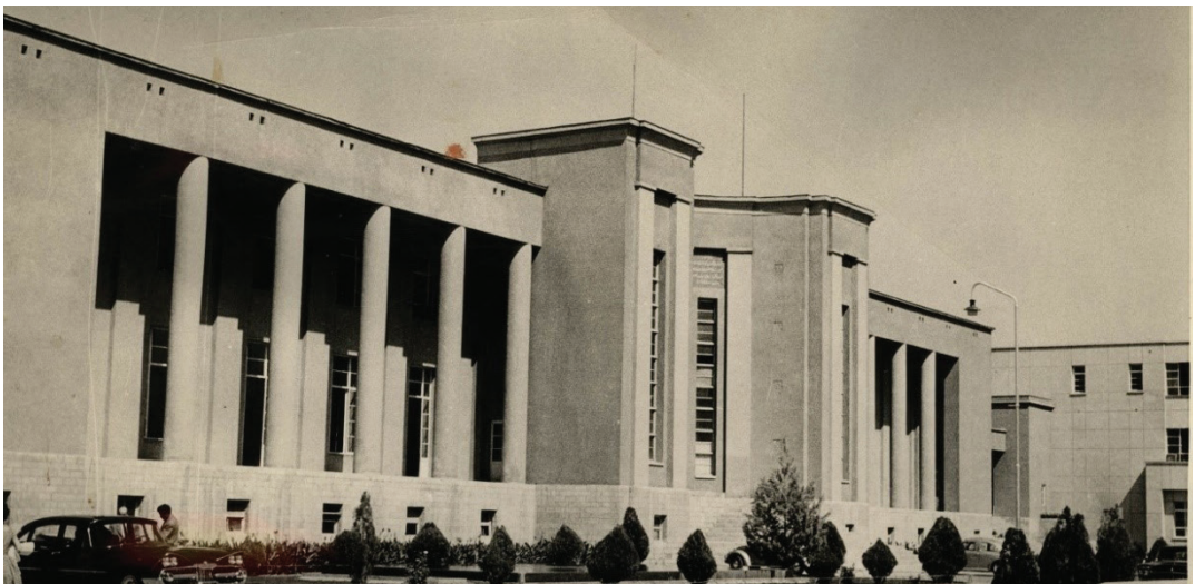
Figure 4. The School of Medicine, general configuration defined by Godard, designed by Maxime Siroux, a Beaux-Arts graduate. (Photograph courtesy of the Central Library of Tehran University, Section of Digital Archive.)
