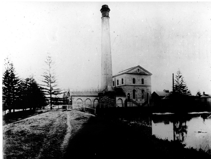
Figure 1. Botany Pumping Station SRC2907, City of Sydney Archives
