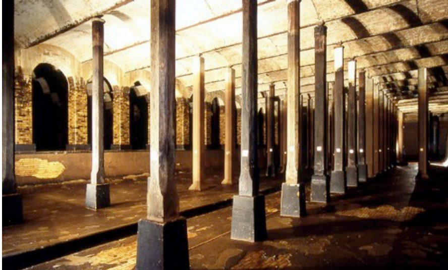
Figure 6. Crown Street Reservoir Sydney Water, 2009.
