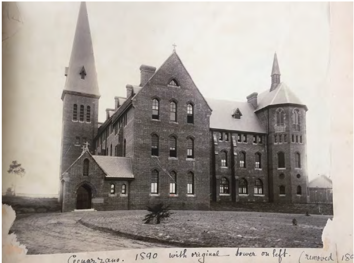
Figure 3. William Wilkinson Wardell, Convent and School as completed. Genazzano, 1890 with original tower on left (removed in 1893). Photograph, Genazzano FCJ College Archives.
