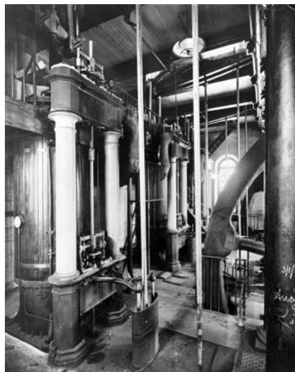
Figure 5. Engines at the Botany Pumping Station. SRC2906, City of Sydney Archives.
