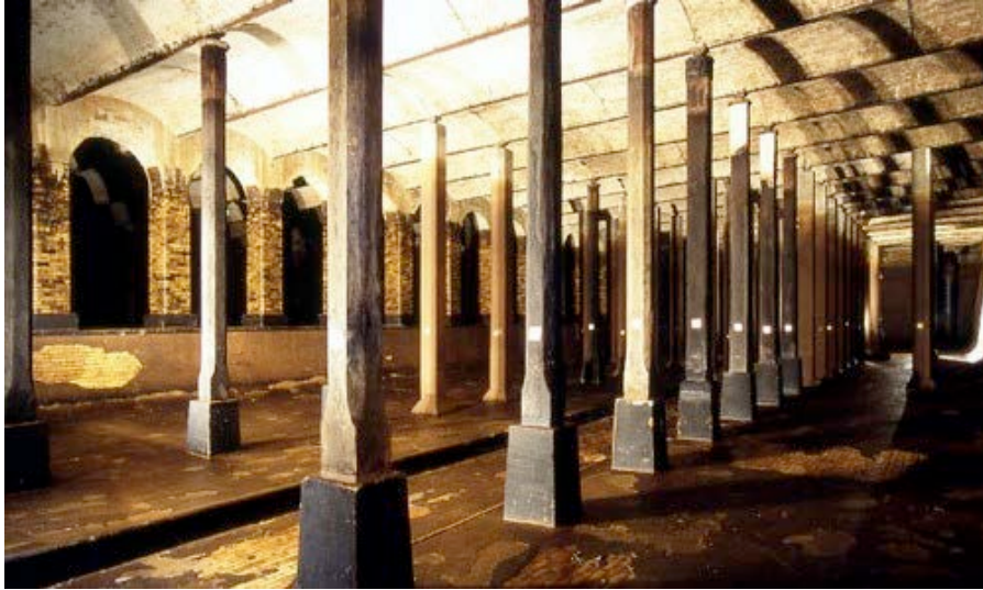
Figure 6. Crown Street Reservoir Sydney Water, 2009.
