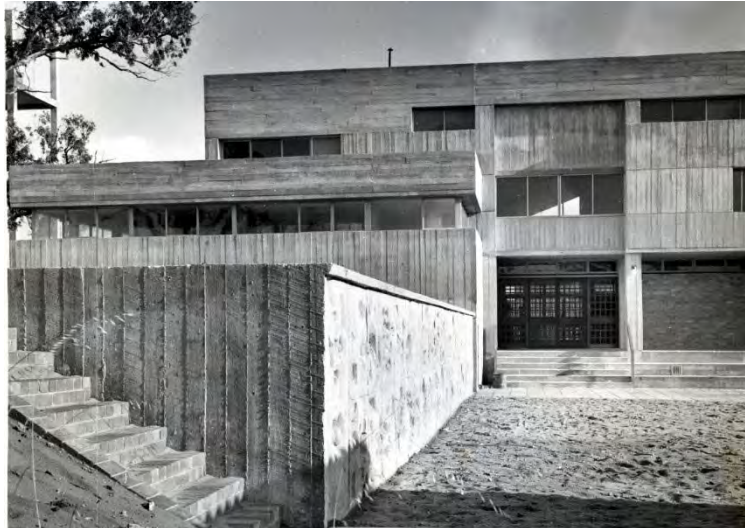
Figure 1: Hale School Memorial Hall, Wembley Downs, 1961.
