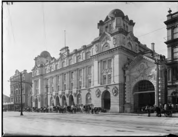
Figure 3. General Post Office, 1912. (Auckland Star: Negatives. Ref: 1/1-002894-G. Alexander Turnbull Library, Wellington, New Zealand. /records/23210653 ).
