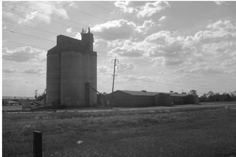
Figure 2. A typical grain elevator, Biloela Queensland. (Photograph by Lloyd Jones, 2017).
