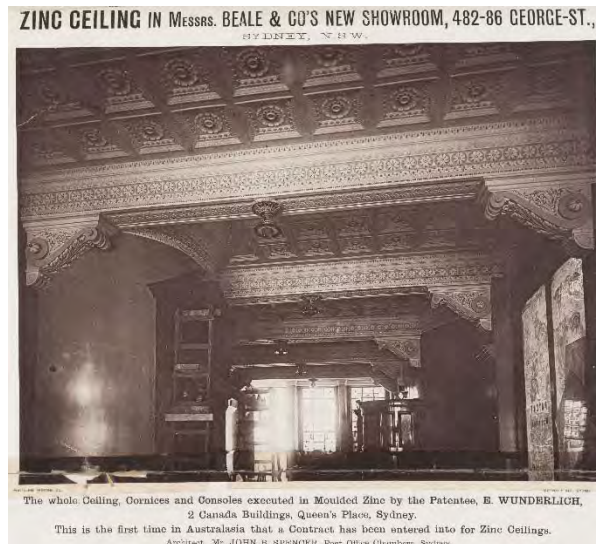
Figure 7. Advertisement for Wunderlich's new moulded zinc ceiling panels ( Australasian Builder and Contractors' News , November 24, 1888, n.p., State Library of New South Wales)
