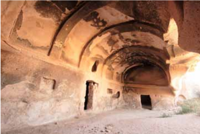
Figure 6: Açksaray. Barrel-vaulted vestibule of Area 5 set parallel to the façade. View towards the northern short wall (photograph by the author, 2011)
