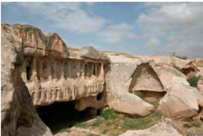
Figure 1: Açıksaray. View of the northwest corner of Area 5 showing the three-sided courtyard, the partly damaged main façade exposing the vestibule behind it, and the partly collapsed kitchen with a conical chimney-vault on the right (photograph by the author, 2012)
