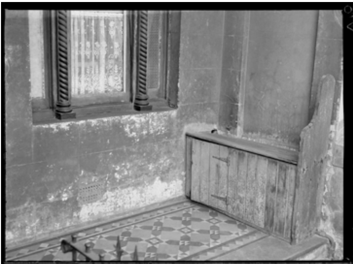
Figure 5. Exterior detail of house in Great Buckingham Street.
