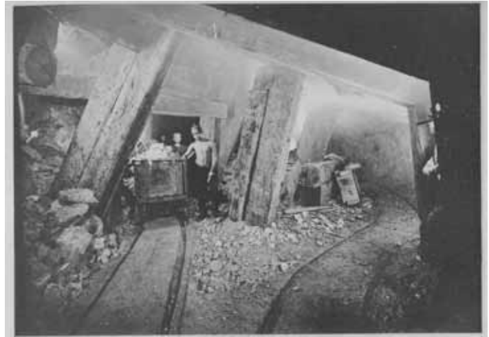
Figure 6. Photograph of Trammers in the New Almaden Mine, 1880s. Trammers pushed and pulled ore carts through the dark tunnels of the mine to the shafts. While many trammers were Swedes, Mexican men also worked tramping ore. Photograph is by Robert Bulmore. (Sullivan and Felton, A Contested Election in California . 1887).
