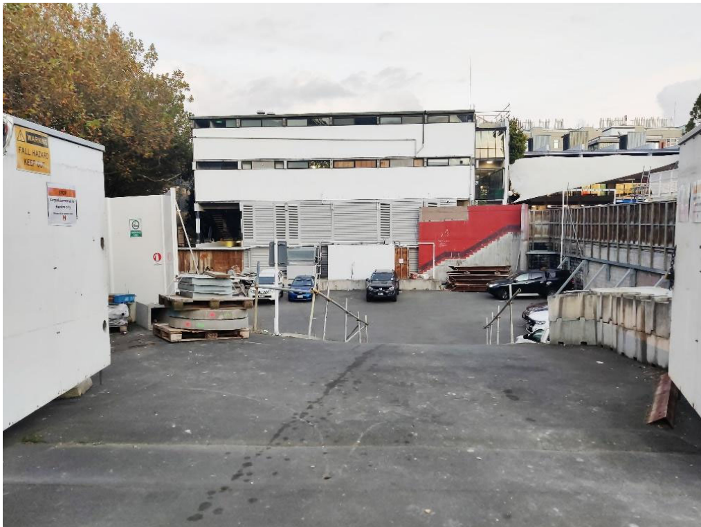
Figure 6. Maidment Theatre demolition plot, 2022 (Candida Rolla).
