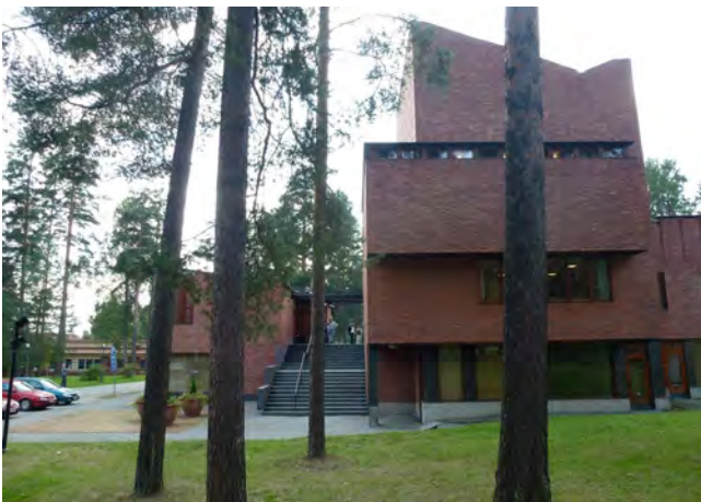
Fig. 1 Säynatsälo Town Hall. Eastern granite stairs and council chamber. Photograph by John Roberts, 2008.
