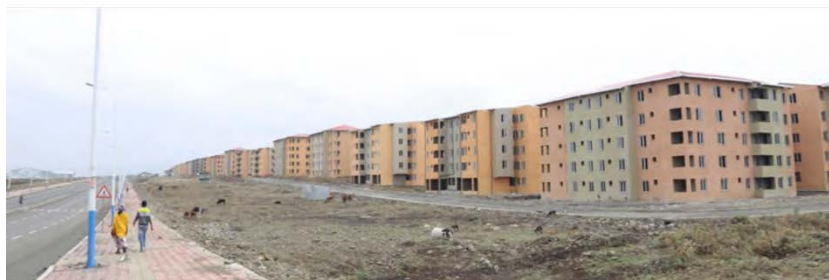
Figure 4. Condominiums built in Koye Feche in the framework of the Integrated Housing Development Program' (IHDP), Addis Ababa, Ethiopia. Source: https://addisfortune.news/amid-tensions-city-identifies-housing-unit-winners/
