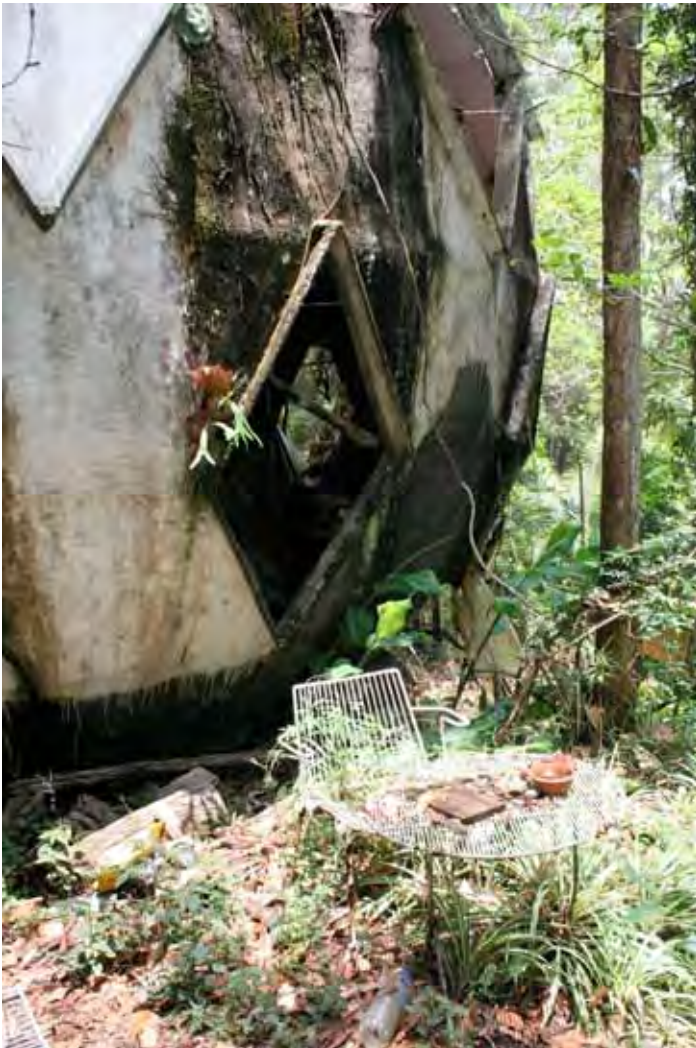
Figure 2. Lee Stickells, 1970s geodesic dome awaiting restoration in northern New South Wales.
