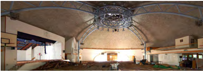
Fig. 5 The binishell at Georges River College, Peakhurst Campus, a few days prior to demolition. Photograph by Alberto Pugnale, May 2014.
