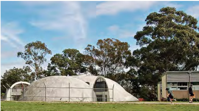
Fig. 3 The binishell at Killarney Heights Primary School is presently used as gymnasium but it suffers from major waterproofing issues. Photograph by Alberto Pugnale, May 2014.
