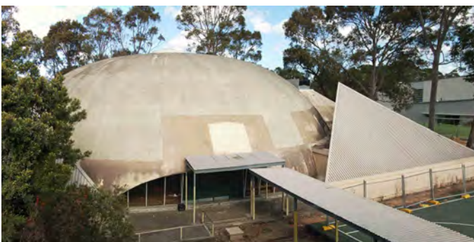
Fig. 4 The binishell at Georges River College, Peakhurst Campus, a few days prior to demolition. Photograph by Alberto Pugnale, May 2014.
