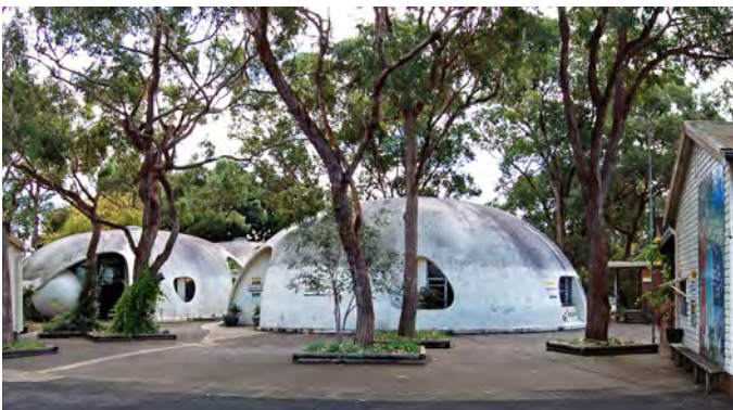
Fig. 1 The three binishells at Narrabeen North Public School. Photograph by Alberto Pugnale, May 2014.
