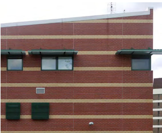
Fig. 5 Detail, Roma Street Fire and Ambulance Station, Brisbane, 2007, Project Services (Design Architect: Spence Jamieson). Photograph by Ashley Paine, 2014.
