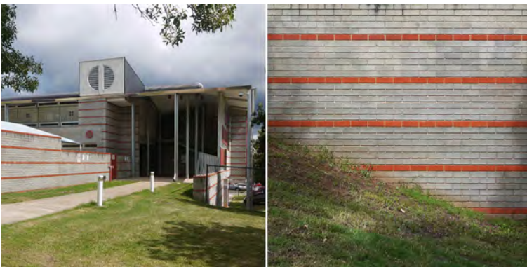
Fig. 2 Street view (l) and (r) detail of Block B, SQIT, Toowoomba, 2002-6, Project Services (Design Architect: Donald Watson). Photographs by Ashley Paine, 2015.
