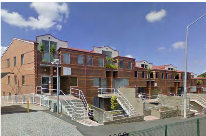
Fig. 1 Southpoint Office Building, Brisbane, 1981-82, Donald Watson (undertaken within the office of Frank Spork & Associates). Image: Google Maps, c. 2010.
