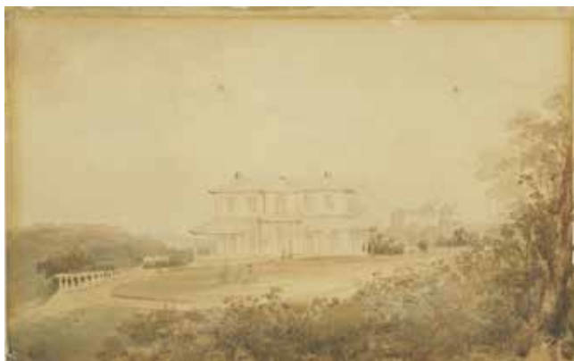
FIGURE 2 Barncleuth, Woolloomooloo, Sydney, 1853 by John W. Brown. (Mitchell Library, State Library of New South Wales).
