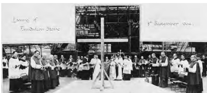
Fig. 2 Archbishop Scanlan laying the foundation stone of St Peter’s before the “entire hierarchy of Scotland”, September 8, 1964. © RCAHMS.
