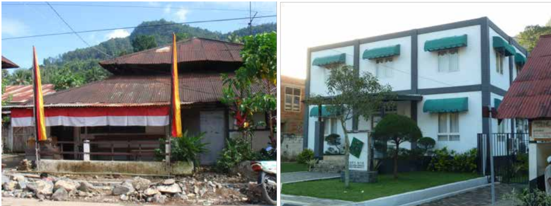
FIGURE 4a The former gathering house for the workers’ association, due to its historical criterion could be valued socially and culturally of significance (left). It was demolished in 2007 to give space for the new Tourist Information Office with its kitsch architecture (right). Source: Martokusumo, 2007 (left) and Martokusumo, 2012 (right)
