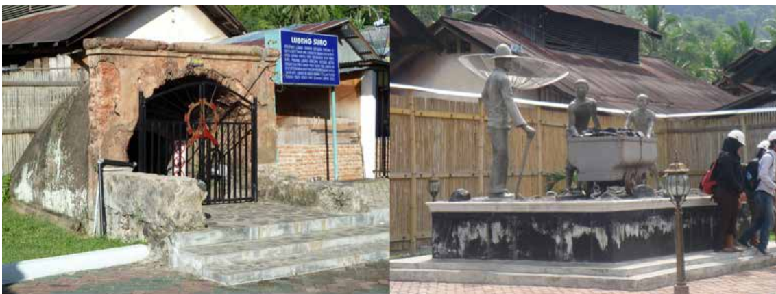
FIGURE 4b The gate of the rehabilitated old tunnel Mbah Suro (left) and the memorial sculpture of mining activity in Sawahlunto (right). Source: Martokusumo 2012, (Left) and Martokusumo, 2009 (right)
