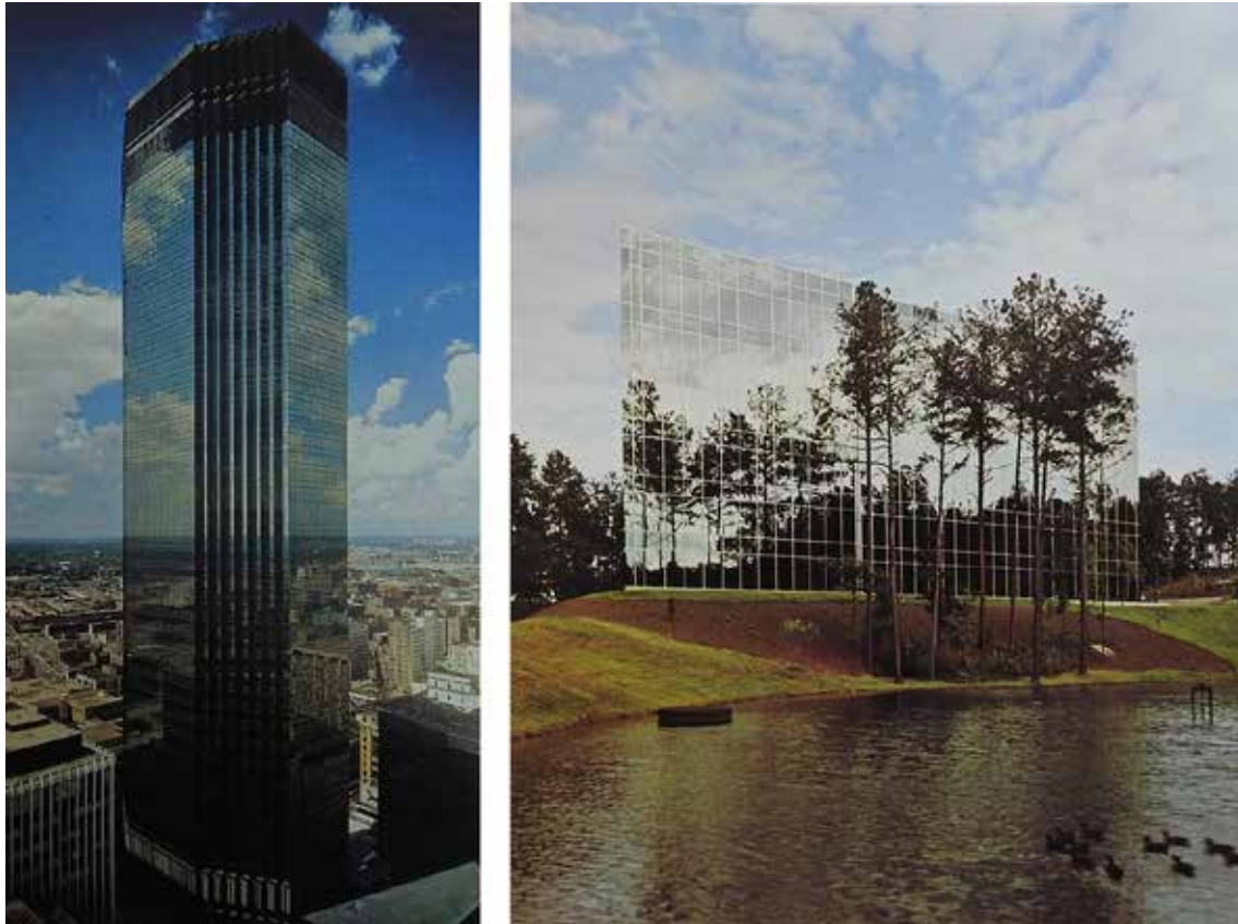
FIGURE 6 All-glass office buildings used to promote reflective glass in America. Left: the IDS Tower, Minneapolis, Johnson and Burgee Architects, 1974. Right: Triangle Building, Atlanta, Thompson, Ventulett and Stainbeck Architects, 1976 (L.O.F. Archives, Canaday Centre, University of Toledo).
