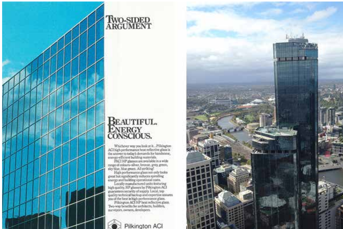
FIGURE 8 Left: reflective glass advertising from Pilkington, 1985 ( Building Product News , August 1985). Right: Rialto Towers, Gerard De Preu in association with Perrott Lyon Mathieson Architects, Melbourne, 1986 (G. Marfella).
