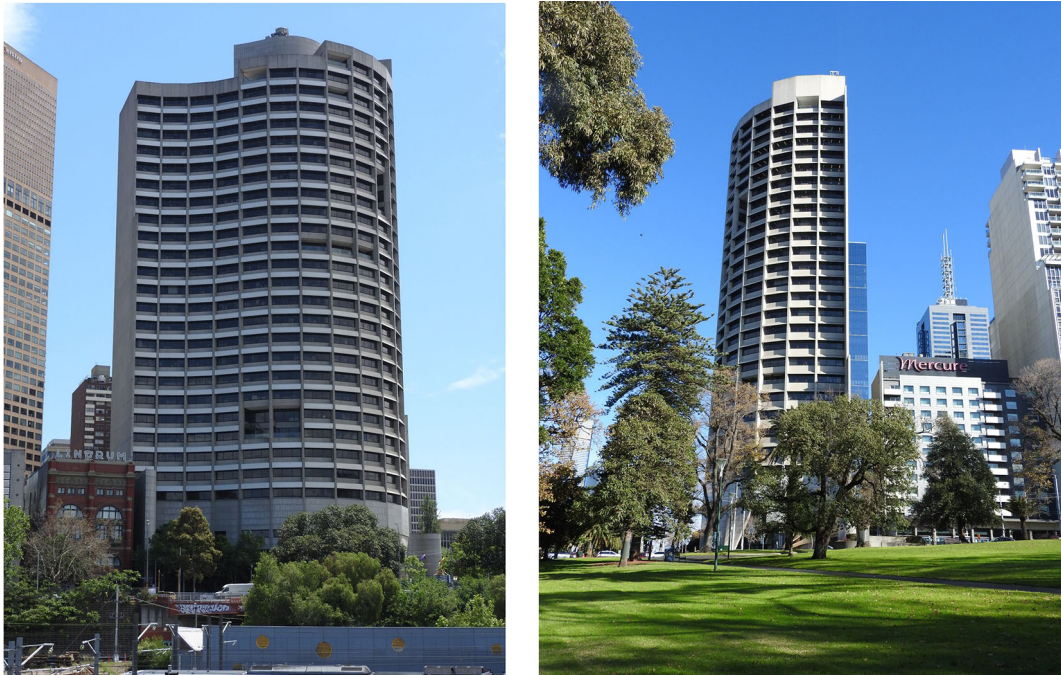
Figure 1. Shell House, 1 Spring Street, Melbourne (1985-88). Architect: Harry Seidler and Associates (Photographs by Giorgio Marfella).
