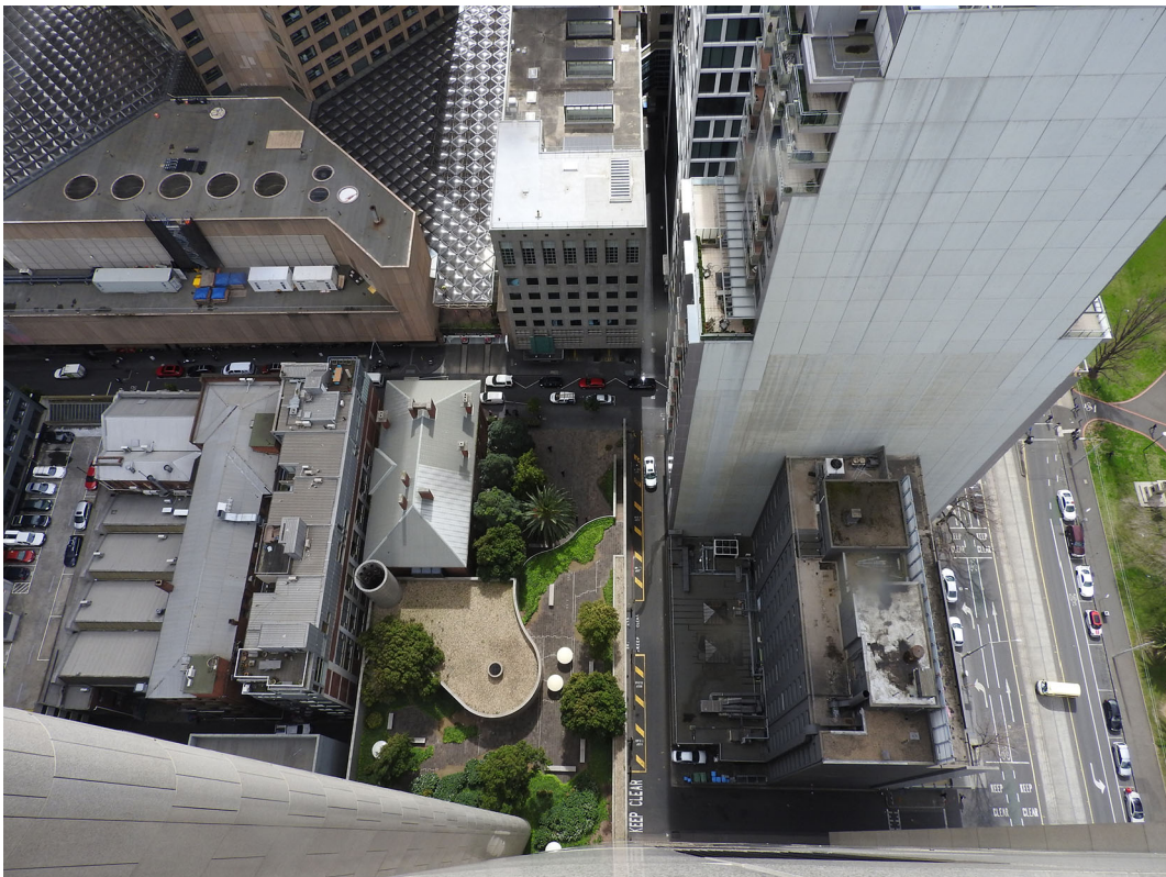
Figure 8. Shell House, Melbourne, view from parapet over Flinders Lane public open space. Architect: Harry Seidler and Associates (Photograph by Giorgio Marfella).
