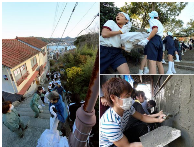
Figure 8. A modern form of yui in Onomichi. Volunteers working together to dispose of waste materials in a relay format and plastering walls during a workshop (Photographs by Onomichi Akiya Saisei Purojekuto).
