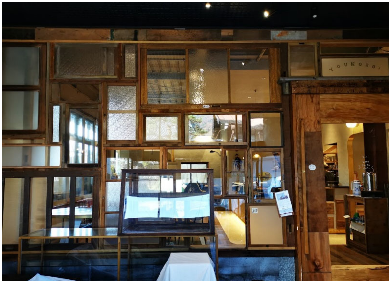
Figure 3. Café entrance at ReBuilding Center Japan. The front of the café is made from repurposed windows and doors (Photograph by Nancy Ji).
