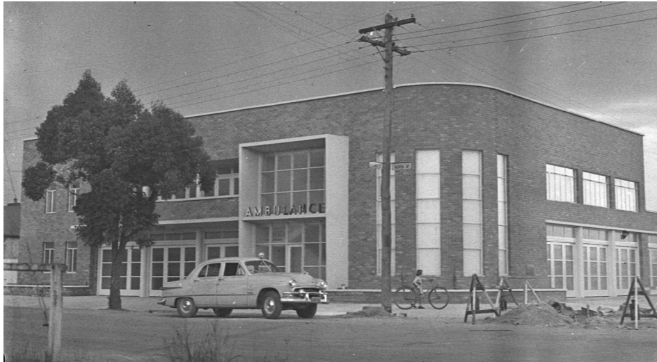
Figure 4. Cessnock Ambulance Station, opened September 1953 (State Library of NSW, Home and Away – 27156, dated 17 September 1953).
