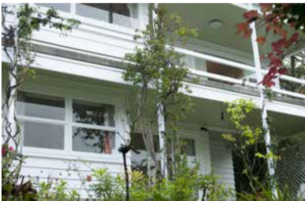
FIGURE 3 Bardwell House, north elevation and verandahs. Source: Photograph by Gina Hochstein, 2016.
