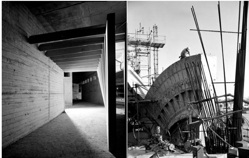
Figure 6. The 'beton brut' finishes of The Sydney Opera House, uncommissioned construction photographs, 1958-1964. (source of images: Mitchell Library, State Library of New South Wales and Courtesy Max Dupain and Associates)
