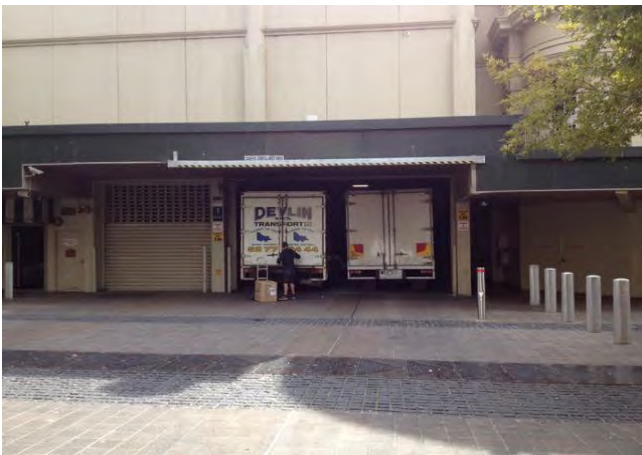
Fig. 5 Loading bay and security grilles to south façade of Market Square Shopping Centre. Photograph by Fiona Gray, 2015.
