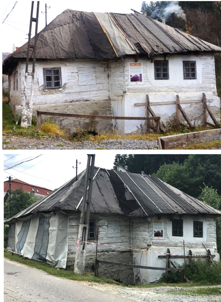
Figure 3. House no. 301. The roof is covered for protection and timber posts support the exterior wall. The finish that has degraded over time is visible around the windows and the base. Top image: 2014, Bottom image: 2017 (Photographs by Alexandra Florea).
