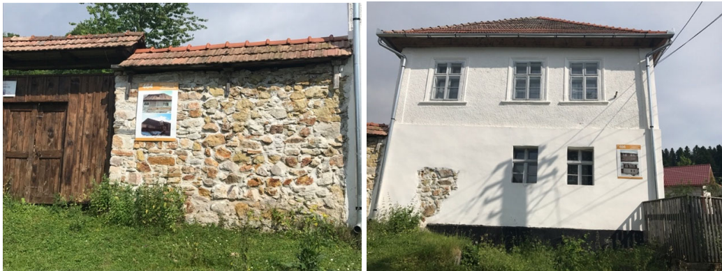
Figure 2. Examples of buildings restored by RMGC (Photographs by Alexandra Florea).
