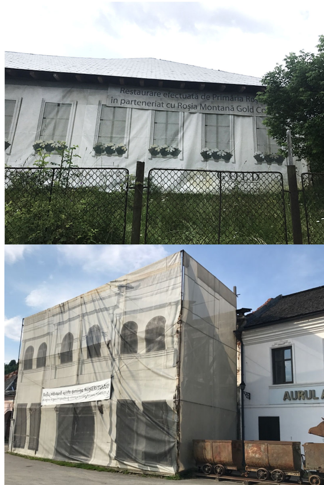
Figure 4. Top image: The message reads: “Rehabilitation by Roșia Montană Town Hall partnered with Roșia Montană Gold Corporation” (tense of the message suggests the rehabilitation has been completed, however in 2017 there was still a canvas to the main façade). Bottom image: “Rosia Montana exists because of MINING! Help us keep a valuable tradition of Apuseni mountains, MINING!” (Photographs by Alexandra Florea).
