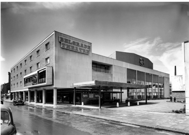
Fig. 1 Belgrade Theatre, Coventry, 1958, Coventry City Architect’s Department. Colin Westwood/RIBA Library Photographs Collection.
