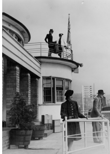
Figure 3. Image of the airport's front façade facing the water ("Rose Bay 1930s," Qantas Heritage Collection).
