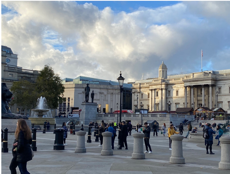
Figure 7. View of National Gallery and the Robert Venturi & Denise Scott Brown-designed Sainsbury Wing (designed 1987) from across Trafalgar Square (Photograph by Robyn Christie, 2022).
