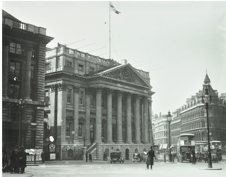
Figure 1. Mansion House in Mansion House Street at the junction of Queen Victoria Street and Poultry, City of London 1930 (© London Metropolitan Archives, City of London, record no. 47771, London County Council Collection).
