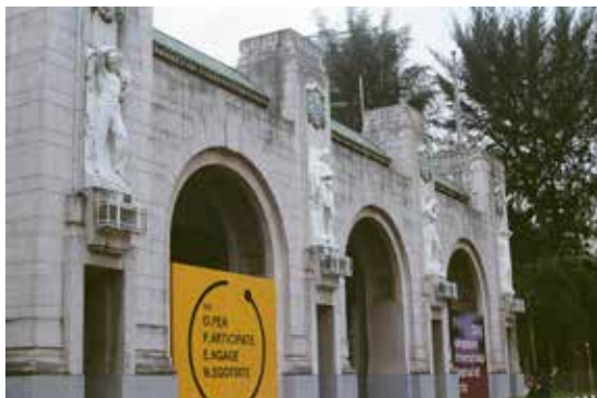
FIGURE 1 Tanjong Pagar Railway Station, entrance portico with marble sculptures and original cast iron lanterns beneath each statue. (Photograph: Liew Yuqi, 2015)
