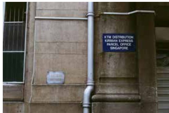
FIGURE 2 Exterior wall rendered in Shanghai plaster, cast iron downpipe and dual language signage. (Photograph: Liew Yuqi, 2015)
