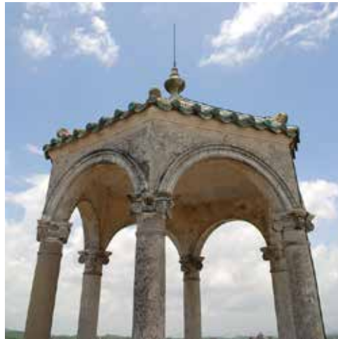
FIGURES 26 & 27 Mingshi Tower, Kaiping
