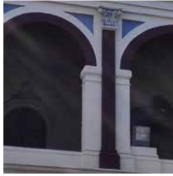
FIGURE 15 Pilaster on the upper level
